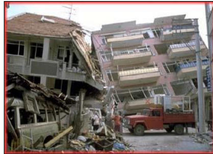
Figure 2: Seismic damage of buildings
